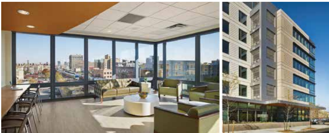
The City used integrated project delivery to build a new hospital wing for NYC Health + Hospitals in under two years.
