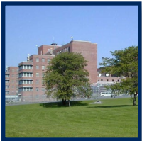
Central NY Psychiatric Center Building 39 & 77 Rehabilitation Jacobs Anticipated Completion: TBD Marcy CENTRAL HEALTHCARE/LIFE SCIENCES
